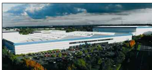
Hozelock's award-winning 33,400 sq m manufacturing and distribution centre is set for years of continual investment
